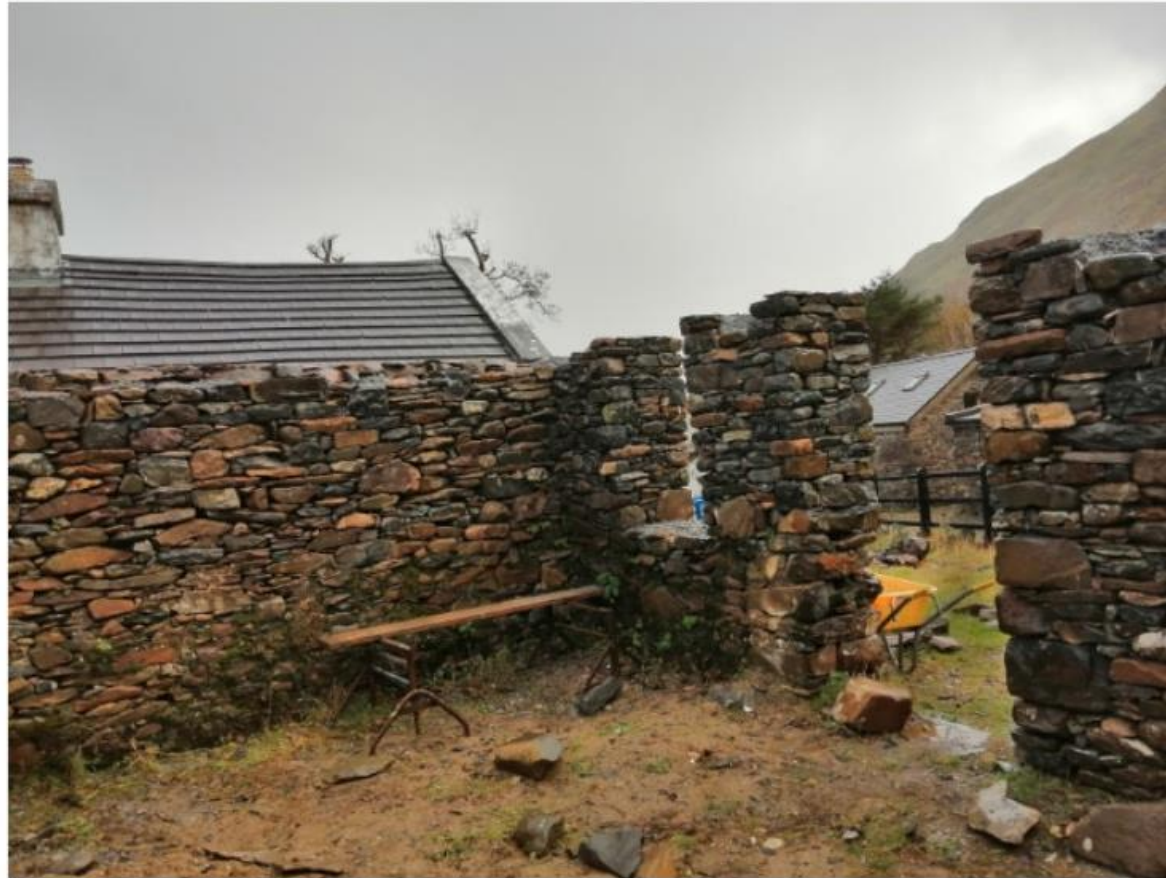
Photo of the cottage walls showing stonework being sensitively repaired in 2021/22.
