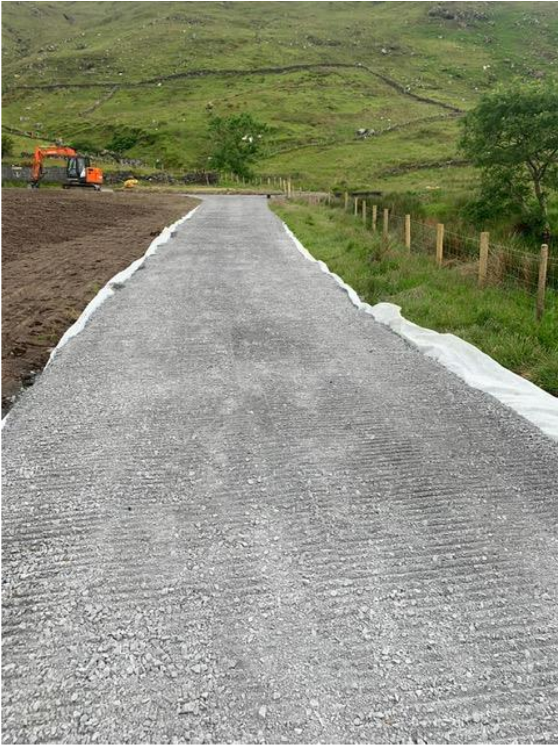
Figure 26. Access track works during the construction phase: terram underlaid and retention of vegetative buffer along the watercourse
