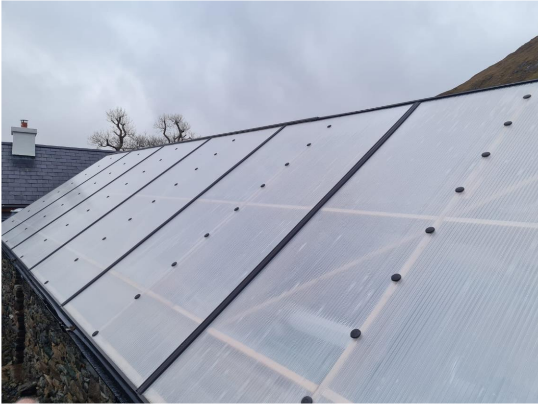
Figure 14. Polycarbonate roof installed on cottage
